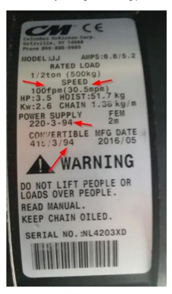
The key items that indicate that this is a 94Hz motor are the fact that the motor is rated at running at 100fpm or 30.5mpm, and the motor Hz is specified at 94
